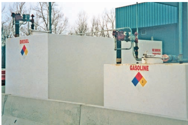
Class I, Gasoline and Diesel Fuel Dispensing
